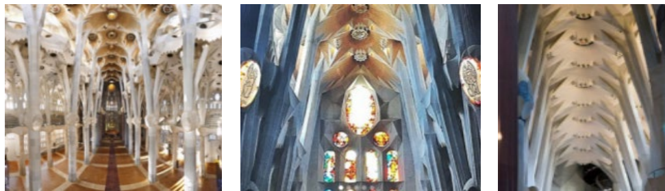
(Fig. 5): Views through arcades: transept, nave, and aisles, [46], and other real by Authors
